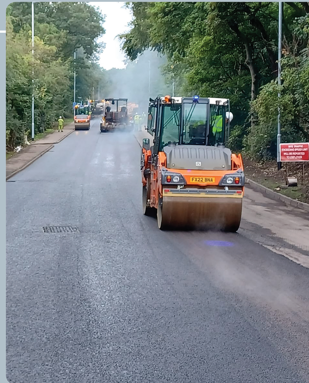
Road resurfacing on Brockholes Brow
